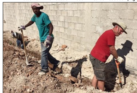
Salem member Tom Marenic (right) works on a footer.
