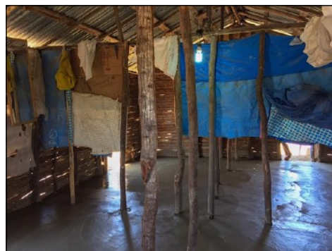
Mission team converts dirt floor to concrete in a home.
