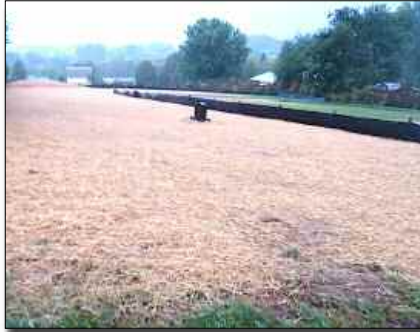
Cemetery rock removal project completed and disturbed area has been seeded.
